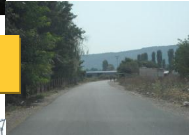
Stacioni i pompave te ujesjellesit Merqi Pumps stacion of water supply Merqi
